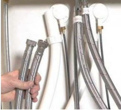
Connect to Shut Off Valves (not included)
